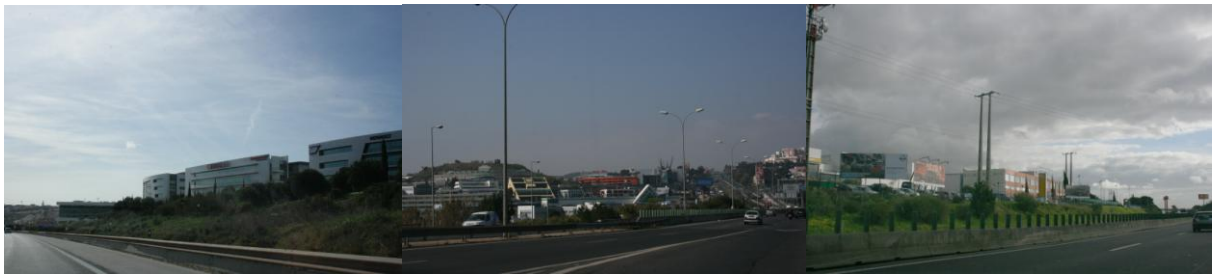
Fig. 2-4: Programmatic specialization areas: Porto Salvo (technological and production); Alfragide (leisure, retail and distribution) and Feijó (production, processing and distribution). Own elaboration, 2012.
